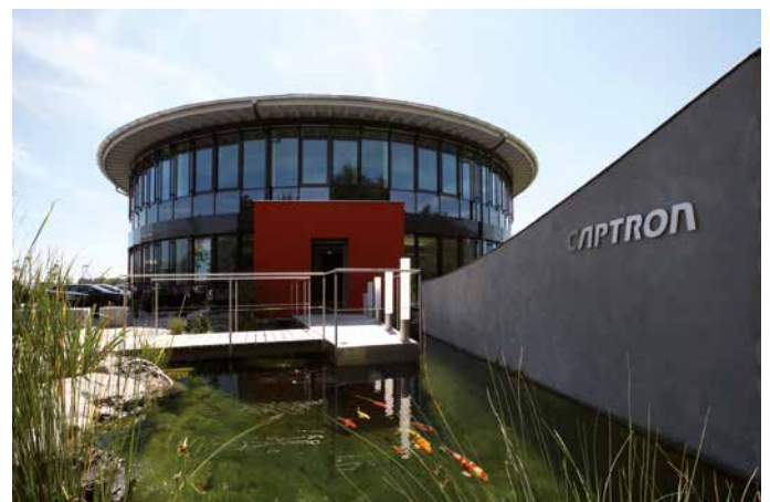
Abb.: Headquarter, Olching - Bavaria
